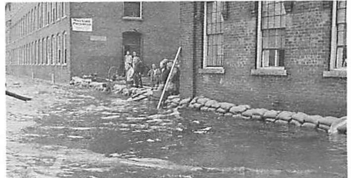
One of the steps in the flood battle was building a sandbag barrier.
